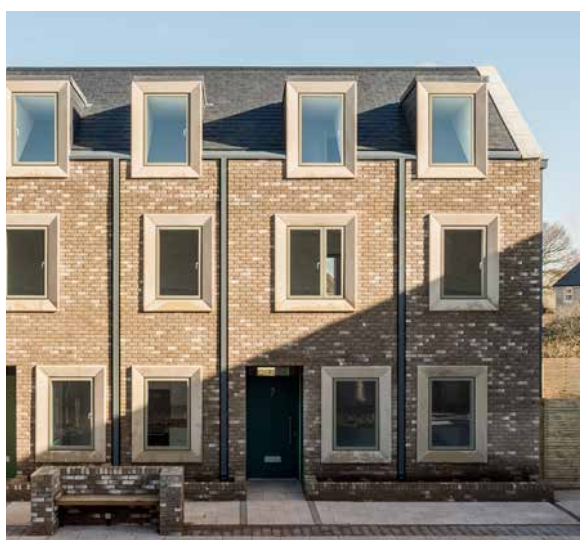
Figure 1.83: Temple Gardens, Temple Cloud, Bristol. Rinterpretation of traditional forms and fenestration with use of traditional brick and stone window surrounds. A design that feels rooted in place without resorting to pastiche. (Archio)
