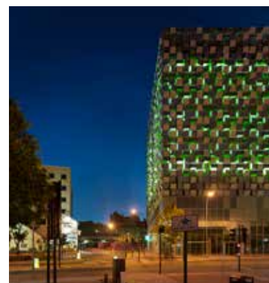
Figure 1.69: The Charles Street multistorey car park in Sheffield creates a striking landmark and helps to define a gateway to Sheffield city centre.
