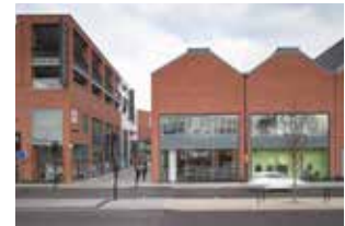
Figure 1.6: Improved road environment at Hereford Old Market
