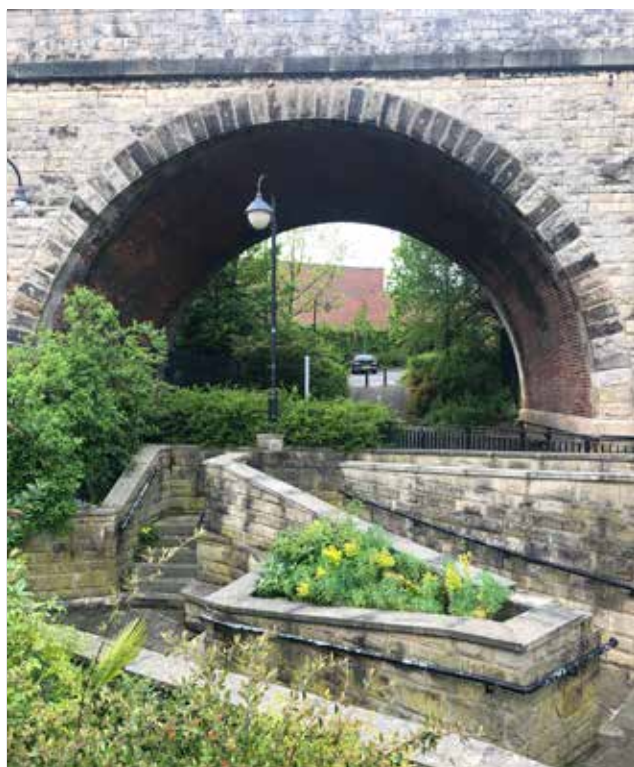
Figure 1.59: Photos of the viaduct
