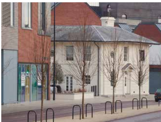
Wide pavements, tree planting and cycle parking in a central reservation show how a busy ring road environment can be transformed at Hereford livestock market
