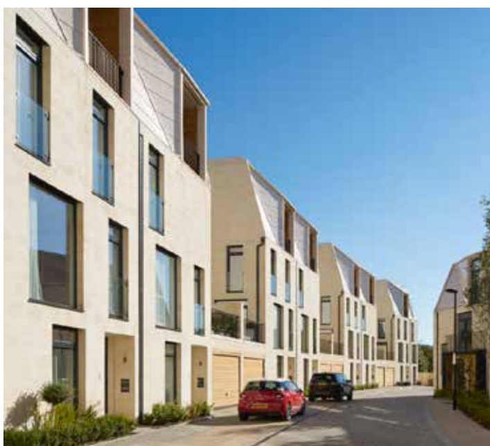
Figure 1.82: A dense four storey typology with use of stone - a modern relation to the rhythm of the regency style with town houses perfect for a historic town centre setting (Alison Brooks Architects)
