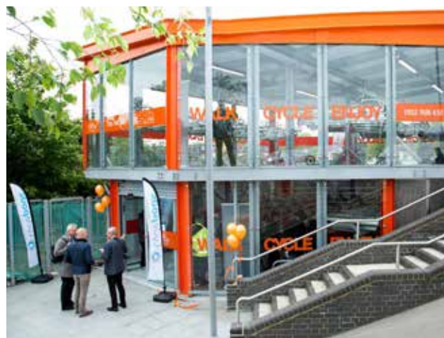
New cycle hubs have been installed at key stations in Waltham Forest. These have CCTV, key fob entry, lighting, tyre pumps and tiered cycle storage. These secure facilities make it easier for people commuting or shopping locally to travel by bike
