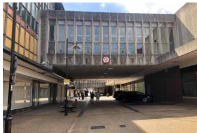
Figure 1.19: Existing Stockwell gate bridges
