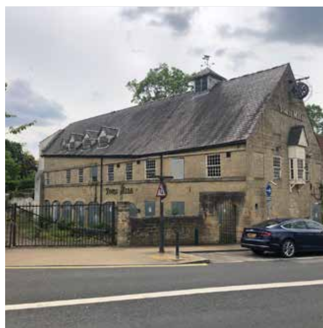
Figure 1.58: Photos of the existing building
