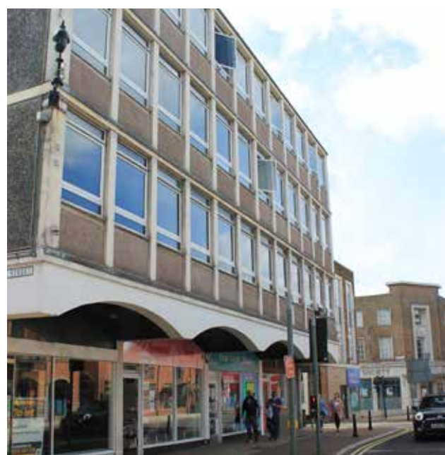
Figure 1.40: Photos of the existing building
