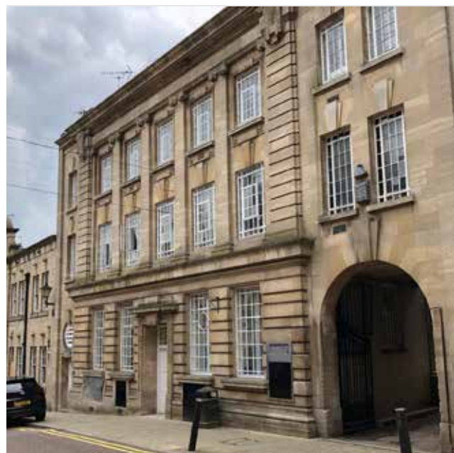
Figure 1.56: Photos of the existing building
