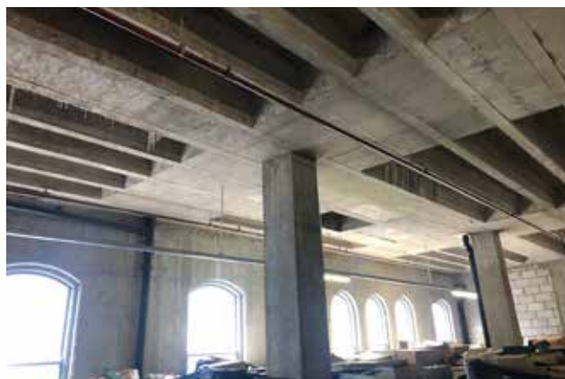
Figure 1.28: Modern structure behind the retained facade
