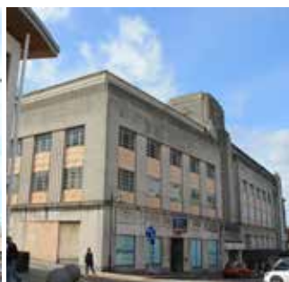
Former Co-op HQ/Beales
