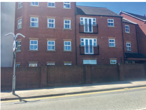
Figure 4.17 Poor relationship between building and street
